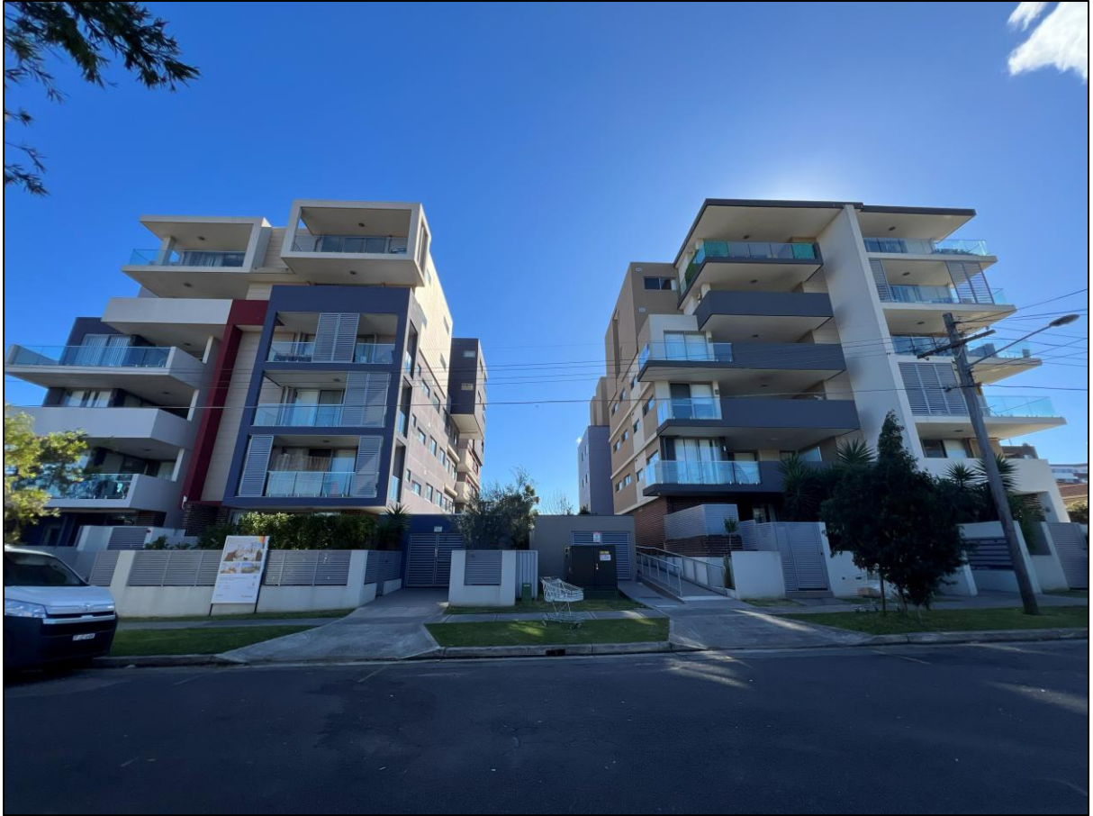
Figure 10. Residential flat buildings at No. 27-37 Percy Street (Source: PPUD, 2026)
